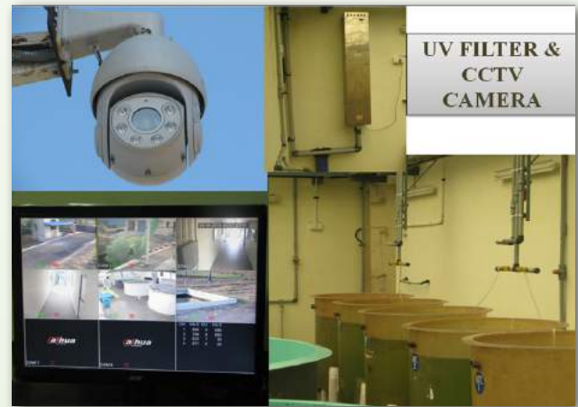
CCTV Camera , UV filtration
