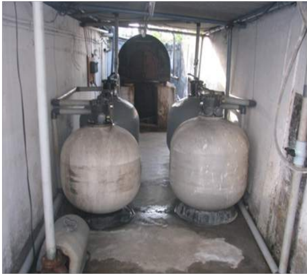
Sand filter system and softner for hardness reduction
