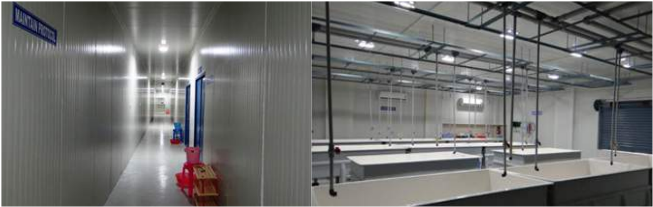
Inside view of second phase of AQF
