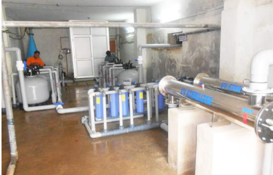
Filtration & seawater treatment equipment
