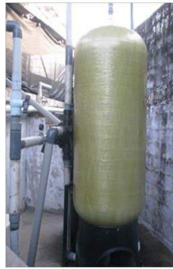
Sand filter system and softner for hardness reduction
